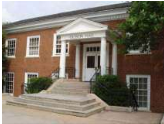
The building where I worked.
